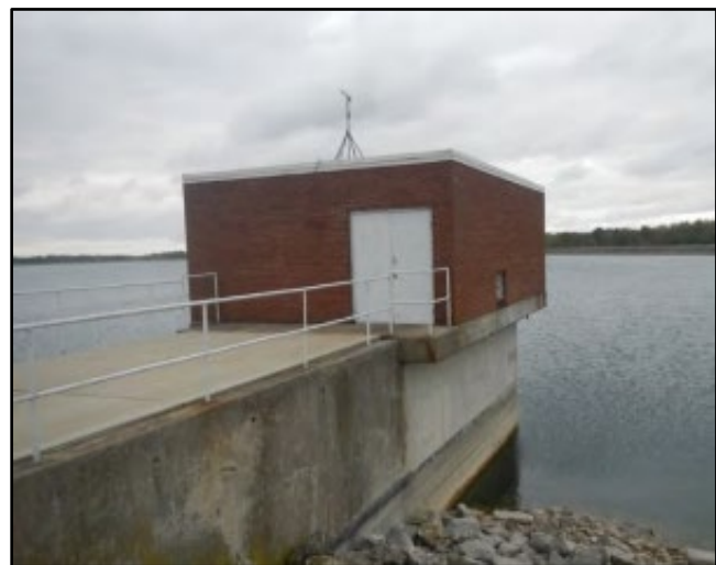
Figure 2. Reservoir intake building
